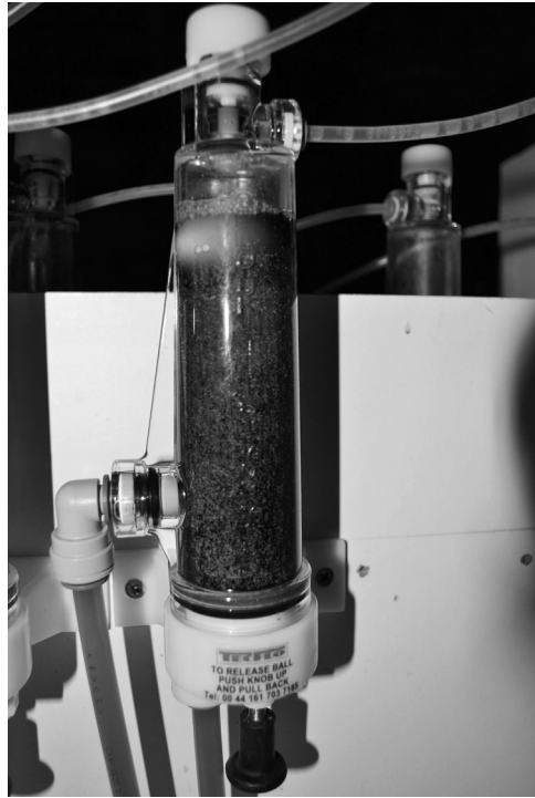
Figure 16.4 Contaminated FOB detector.
